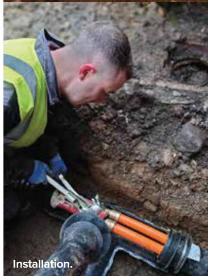
Heating pipes at Penicuik Estate.
