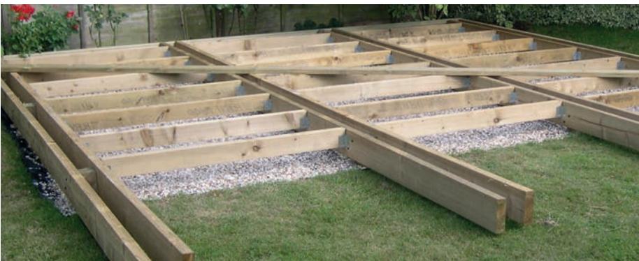
Supplying a treated wood product like this with a third-party quality accreditation will build buyer confidence and lead to growth in demand
