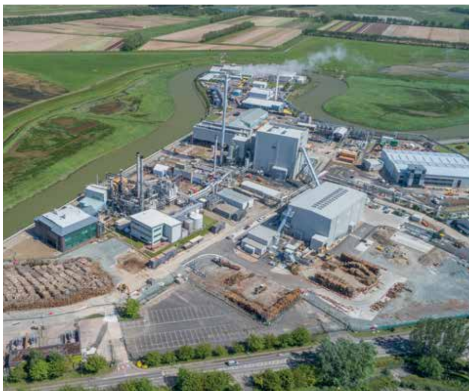
Kent Renewable Energy's CHP plant at Sandwich, Kent, during its last phase of construction in May 2018.
