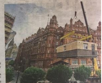
▲ Modular like homes are bolted together on site in Manchester after being transported by lorry from the factory in Knaresborough. Eight houses a day will be produced, fully fitted with
