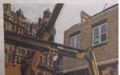
▲ Modular like homes are bolted together on site in Manchester after being transported by lorry from the factory in Knaresborough. Eight houses a day will be produced, fully fitted with
