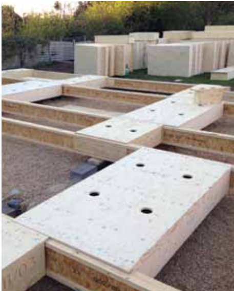
Chassis ground floor by Facit Homes
