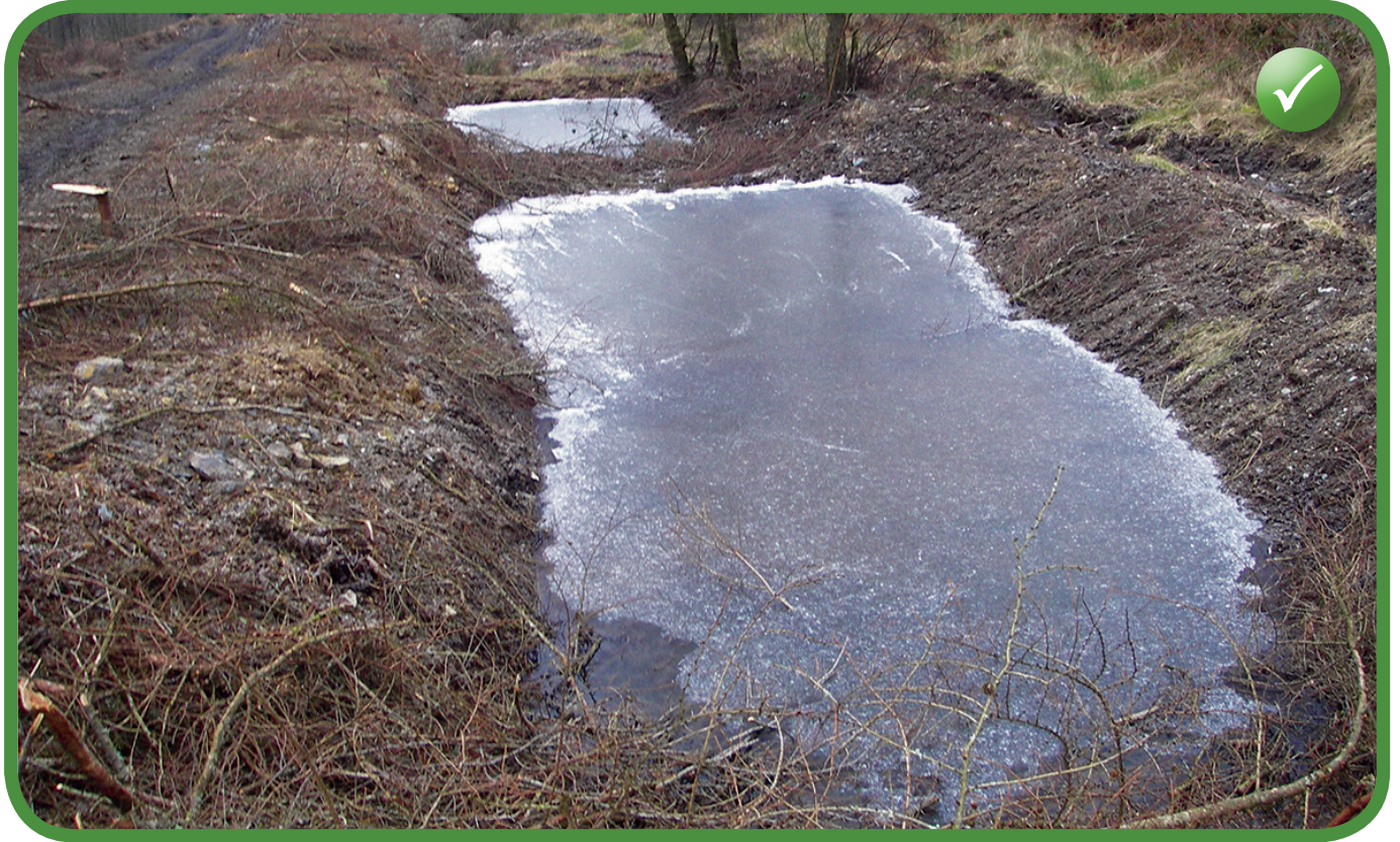
Forwarder Track Settlement sumps in series
