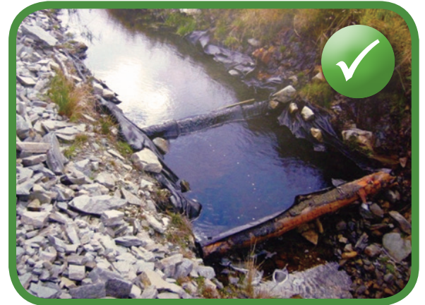
Silt trap / sump with sloping (not flat) bottom
