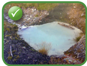
Runoff treatment sump overflow to vegetation
