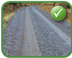
Good quality forest road - no chained vehicles, just lorries travelling on it
