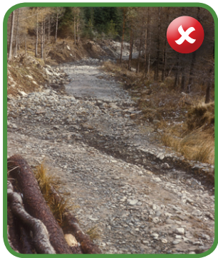
Water making its way across a road
