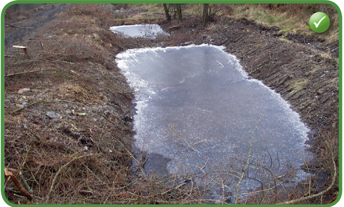
Forwarder Track Settlement sumps in series
