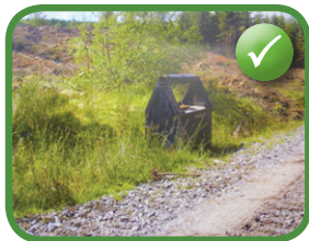
Fuel store on level ground away from drains
