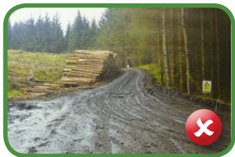
Deteriorating forest road
