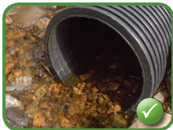
Good practice - culvert
