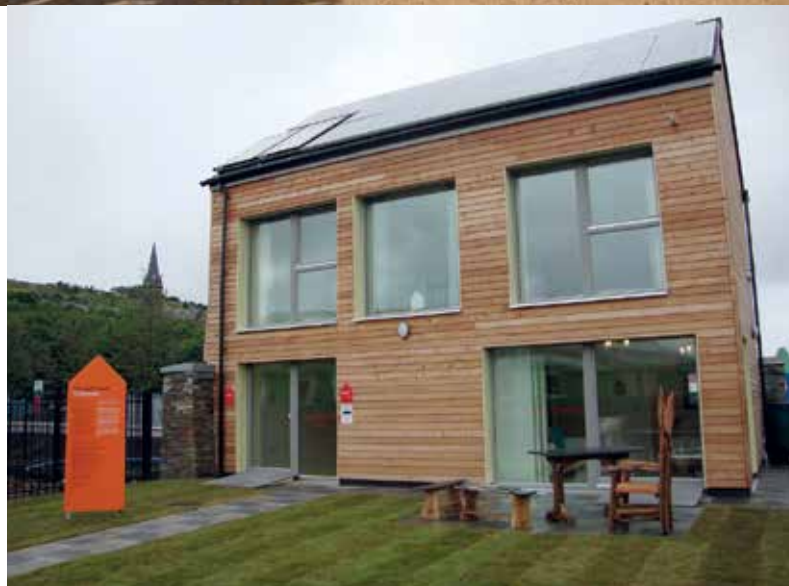
Larch House. Photo credit: G. Pargeter
