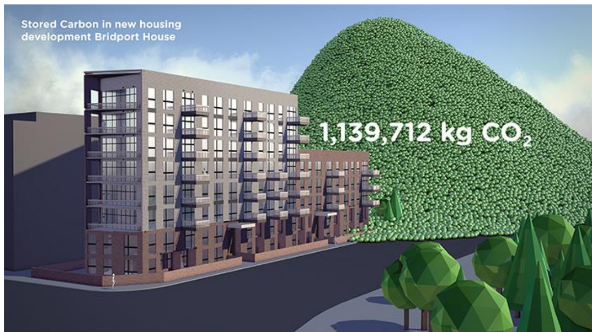
Figure 7. Carbon stored in the Cross-Laminated Timber building Bridport House, Hackney, London which comprises 41 flats. The building used 1,576m 3 CLT which if produced in Wales would require around 7 hectares of forest. Image: Wood for Good.
