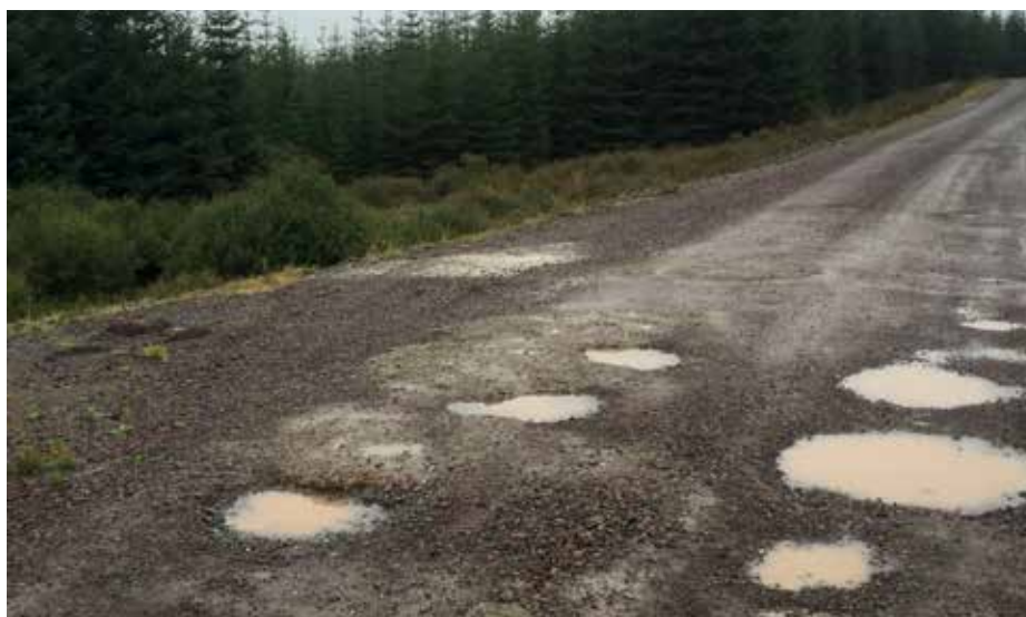
Potholes in a forest road
