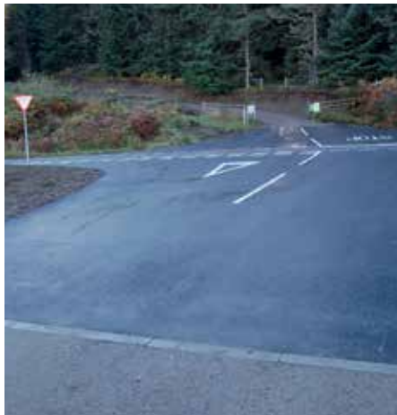
High specification junction between a public road and a high volume shared-use forest road
