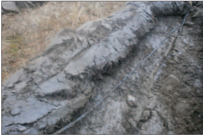
Above: The 50v telecommunications cable pulled up by the plough. You can clearly see how shallow the cable was buried.
