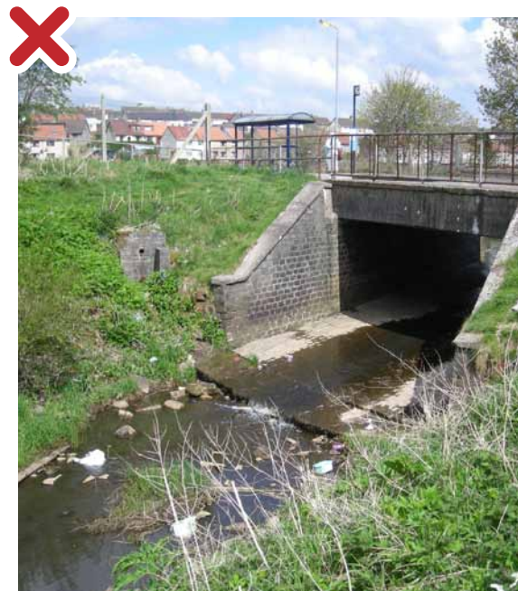
Figure 4: Poor practice. A bridge invert may be level with the riverbed at the time of construction but subsequent erosion downstream due to scour can lead to a drop forming (perched invert) that can create a barrier to fish passage, it can also lead to flows that are too shallow for fish to swim through.
