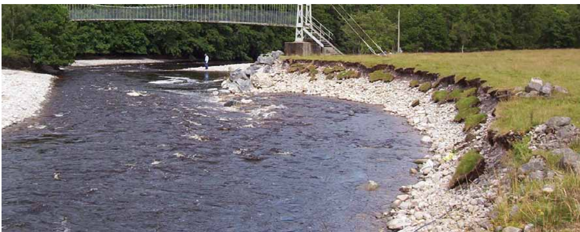
Figure 14: Bridge structure at risk of failing due to erosion from inappropriate location on an active river.
