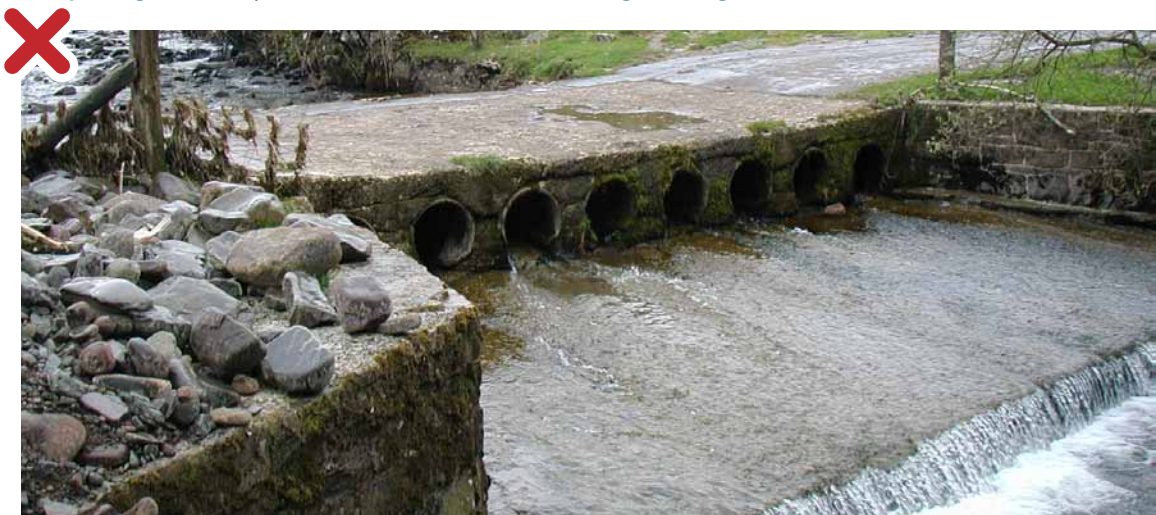
Figure 51: Poor practice, this is not a ford! Fords should not be above the river bed level and multiple pipes should not be used. This creates a barrier to fish passage and can prevent sediment being transported downstream. Raising the ford above bed level increases the risk of bed erosion downstream during high flows this can lead to a drop forming which creates further problems for fish passage and may lead to the need for further engineering.
