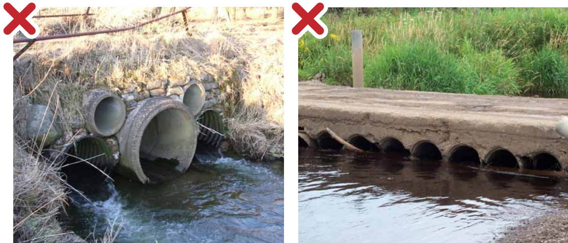
Figure 43: Twin barrel culvert that maintains natural channel width and invert buried below the natural bed level. Should only be used where single span structure or single barrel culvert is not possible.
