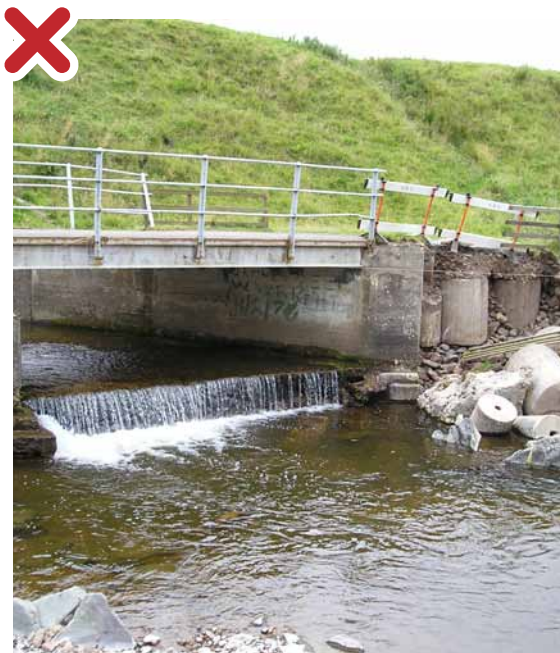
Figure 4: Poor practice. A bridge invert may be level with the riverbed at the time of construction but subsequent erosion downstream due to scour can lead to a drop forming (perched invert) that can create a barrier to fish passage, it can also lead to flows that are too shallow for fish to swim through.
