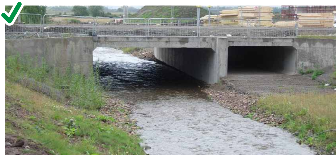
Figure 38: Good practice, culvert maintaining natural channel width, bed level and slope ensuring adequate water depth and water velocity for fish passage.
