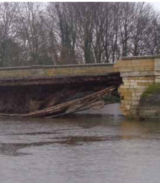
One of the iconic images of the December floods: the collapsed Tadcaster Bridge. (Picture: Mtaylor848)
